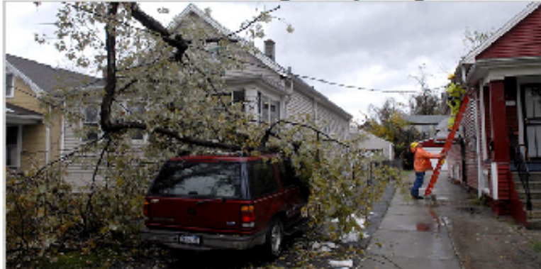
Electrical service workers in Buffalo, N.Y., on October 17, 2006. Mike Groll for The New York Times
